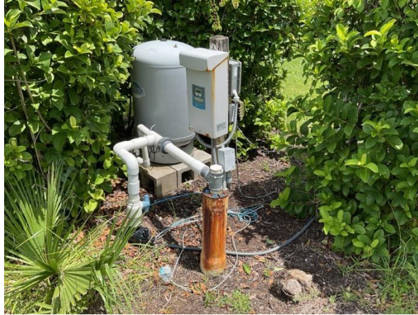
Irrigation system pump
