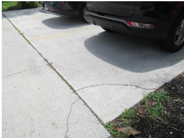
Concrete cracks
